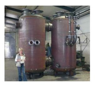
Tanks with 12,000 litres and four dual-circuit evaporators, connected to 8 refrigeration systems, for the catering company of Emirates, Dubai airport. A similar plant has been installed in Frankfurt for the catering company – Lufthansa Sky Chefs.
